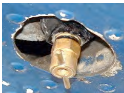
Main Tank Drain
