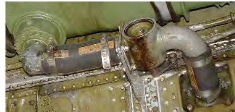
Oil Shutoff Valve
